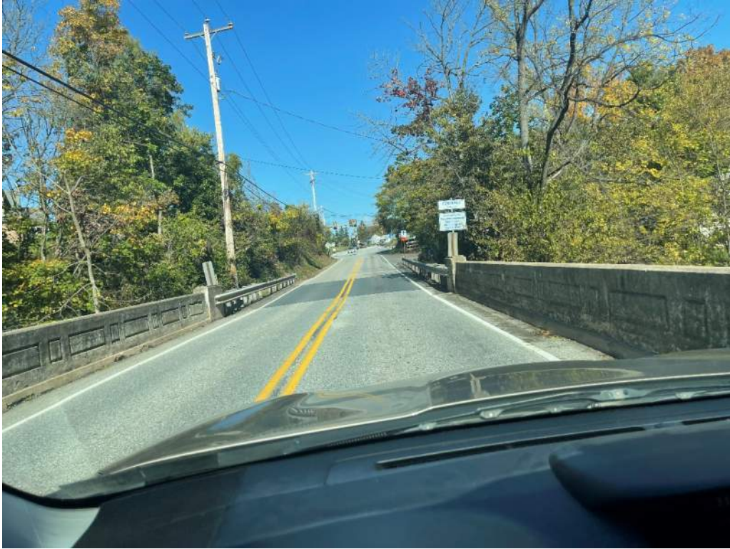
Canal Road (SR 921) and Susquehanna Trail (SR 297) – Northbound Approach
