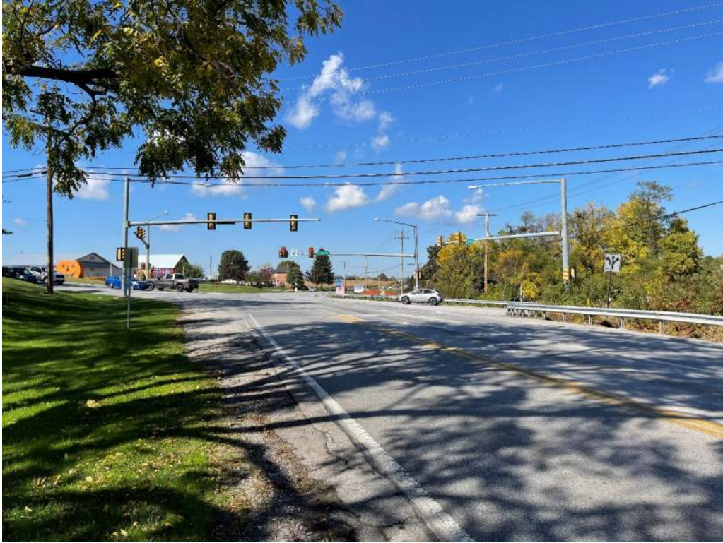
Bull Road (SR 4001) and Church Road – Northbound Approach
