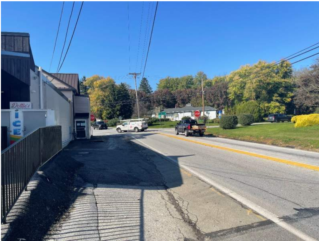
Bull Road (SR 4001) and Canal Road (SR 921) – Westbound Approach
