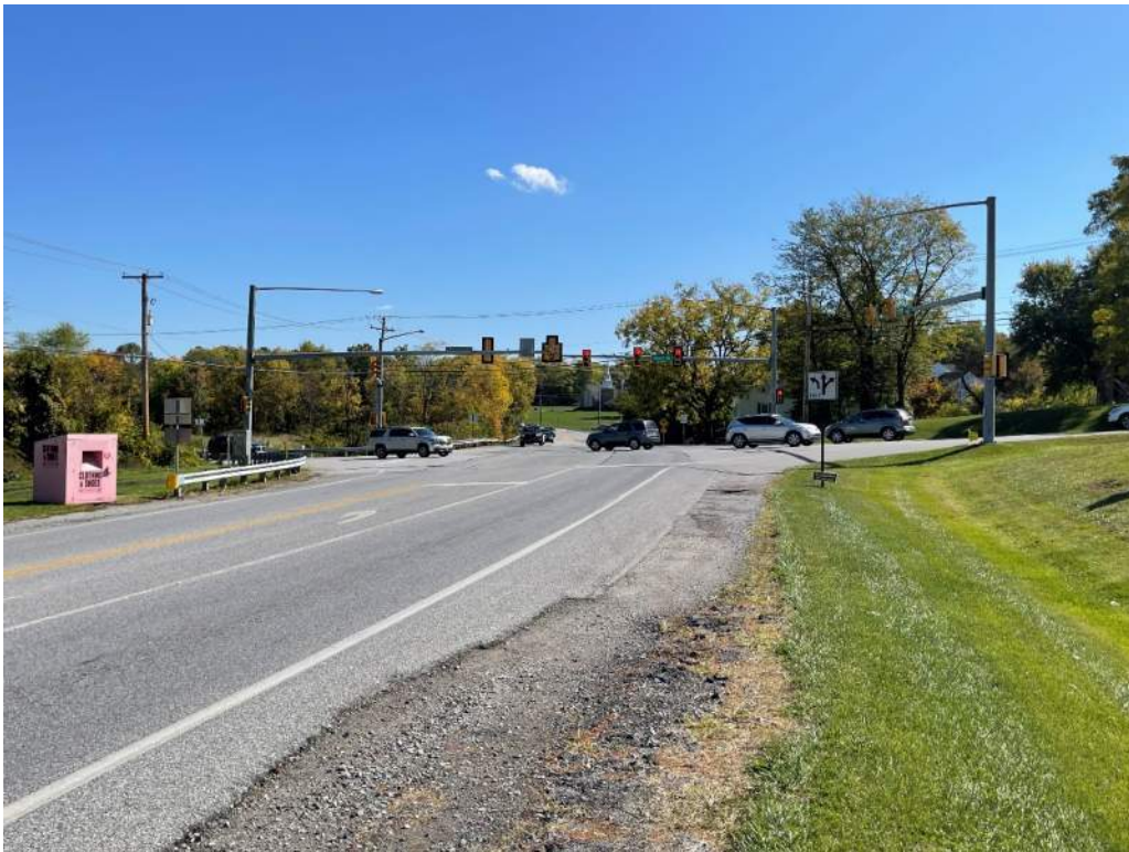
Bull Road (SR 4001) and Church Road – Southbound Approach
