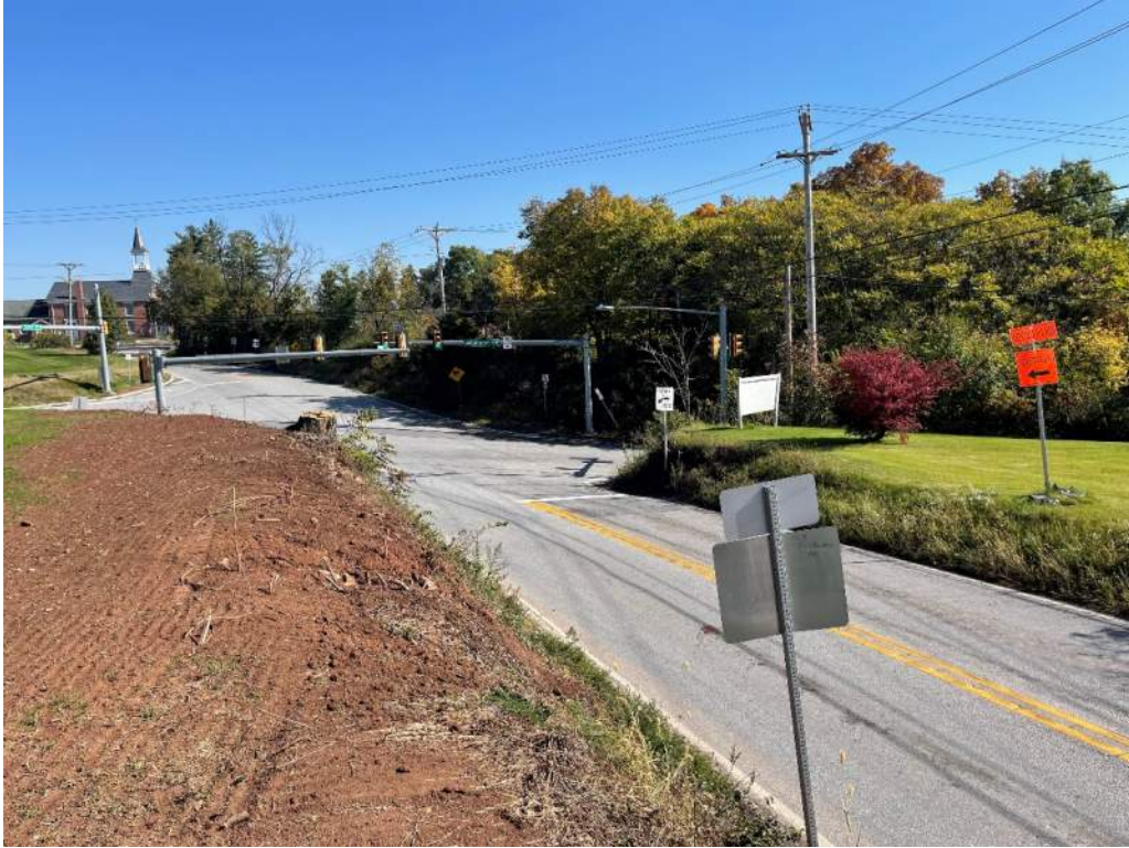
Canal Road (SR 921) and Susquehanna Trail (SR 297) – Eastbound Approach
