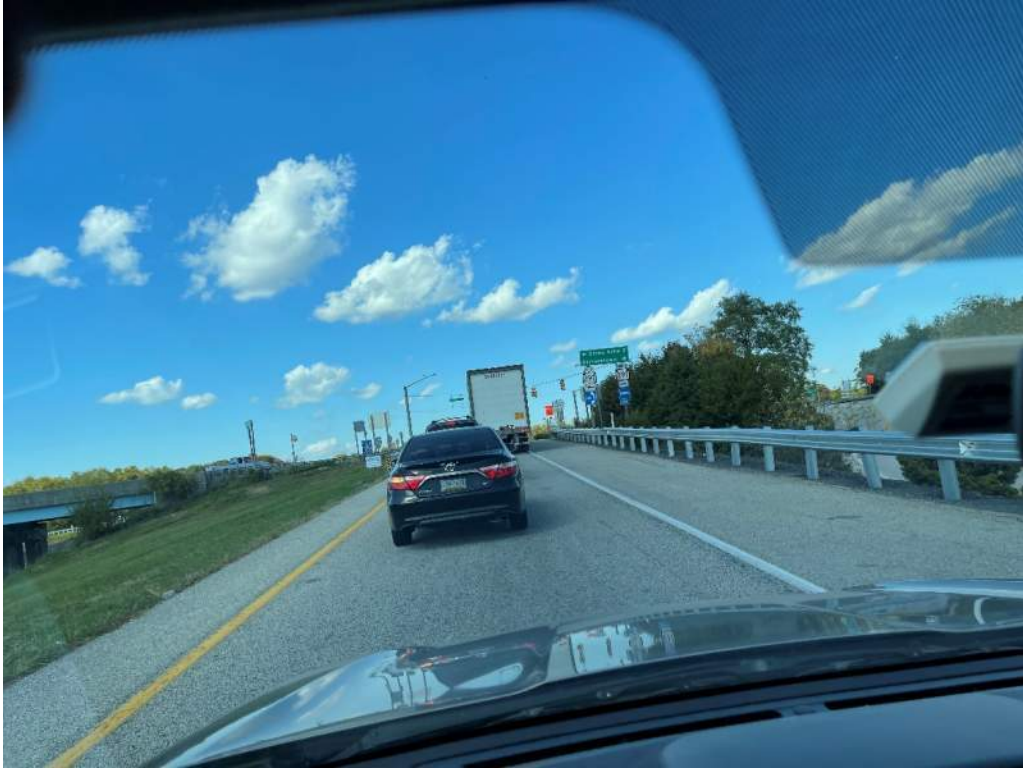
I-83 NB and Susquehanna Trail (SR 297) – Northbound Approach
