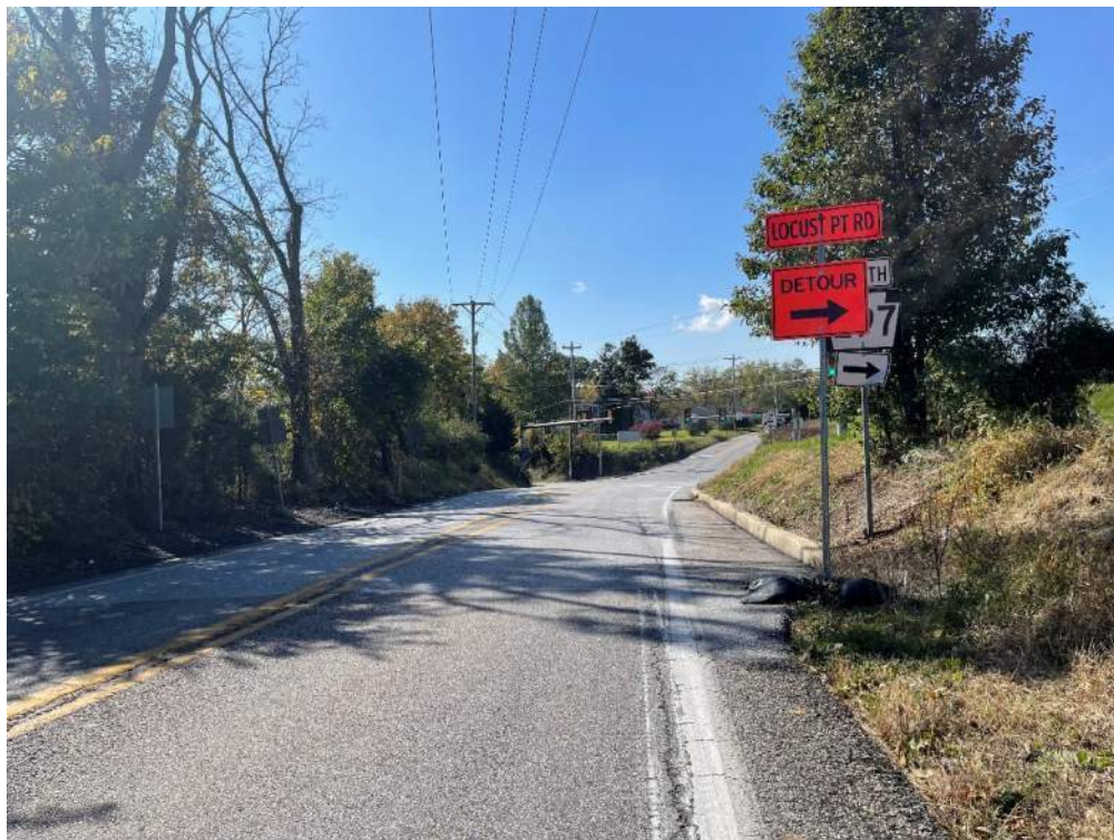
Canal Road (SR 921) and Susquehanna Trail (SR 297) – Westbound Approach
