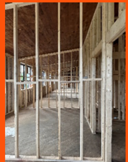
Image 2: Framing on the interior of the existing building.
